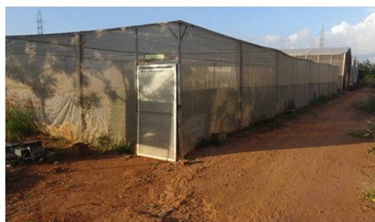
Transgenic containment, nethouse
